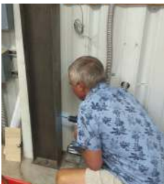
Ed Campau doing metal work prep for wall panel
